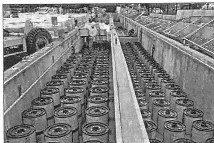
Custom PerkFilter vault in Redmond, WA
