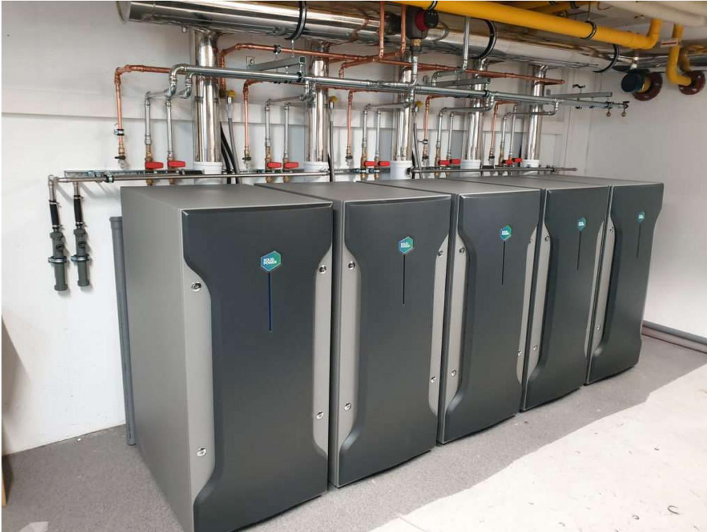
Photo illustrates modularity when the units are manifolded
