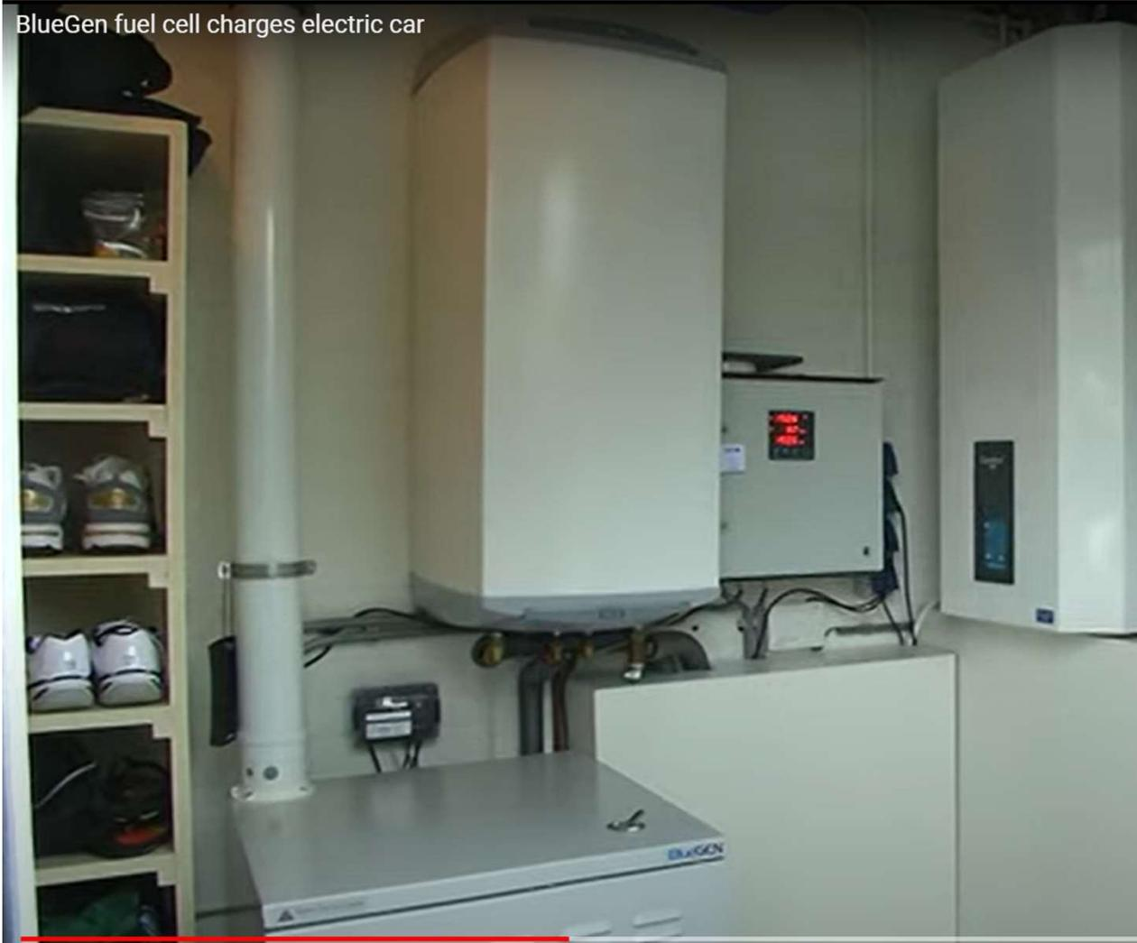
Note: This image from a YouTube video published in 2013, showing the BlueGEN fuel cell powering the home and an electric vehicle, with by-product heat. (ahead of its time)
