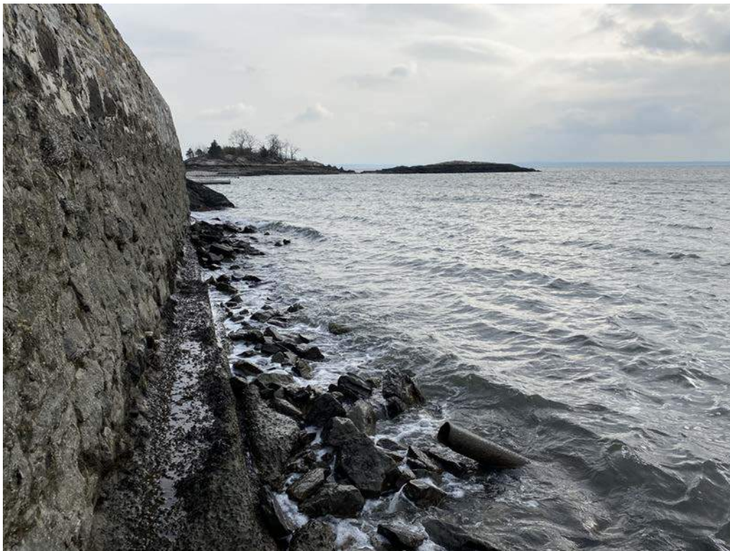
Figure 4: Waterward Face of Wall, Rip Rap Toe Protection Looking Southeast, 12/9/2020
