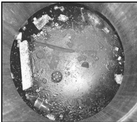
Floatable debris in the Aqua-Swirl®
