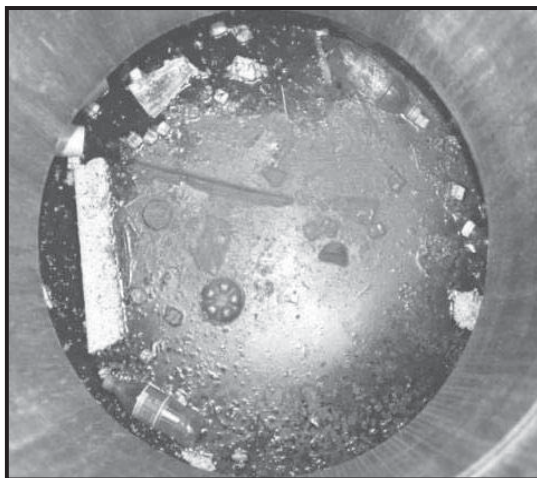
Floatable debris in the Aqua-Swirl®
