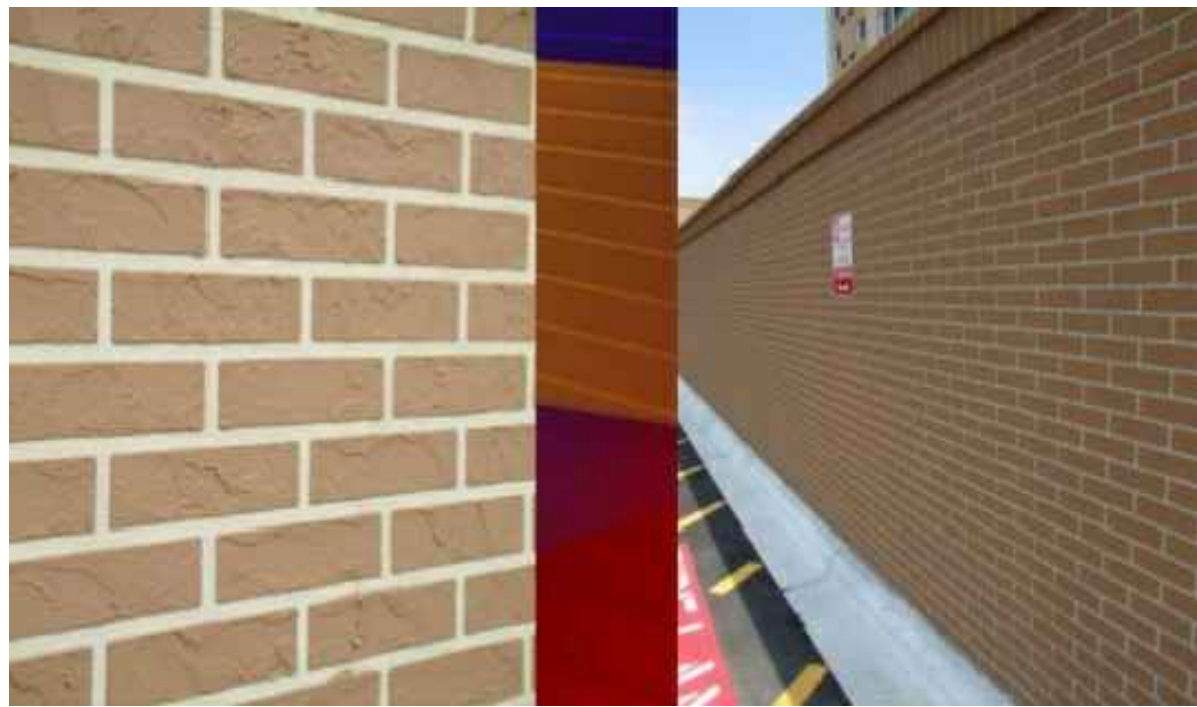
5C EFIS BRICK FACADE DRYVIT
