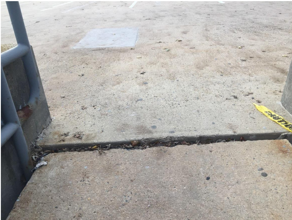
Photo 8: Gap between north stair and slab.
