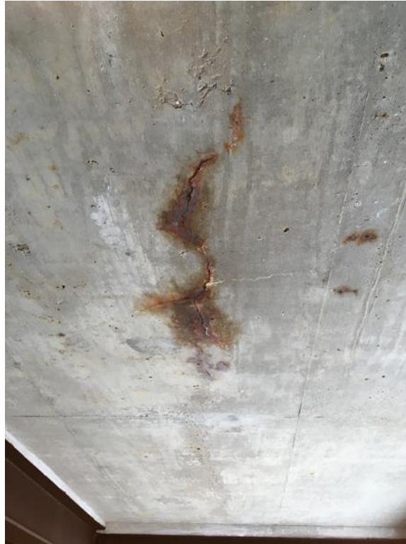
Photo 1: Distressed concrete overhead at slab.
