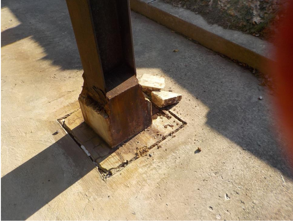
Photo 9: Spalled concrete column encasement with fallen loose concrete. Photo taken at column along south elevation.
