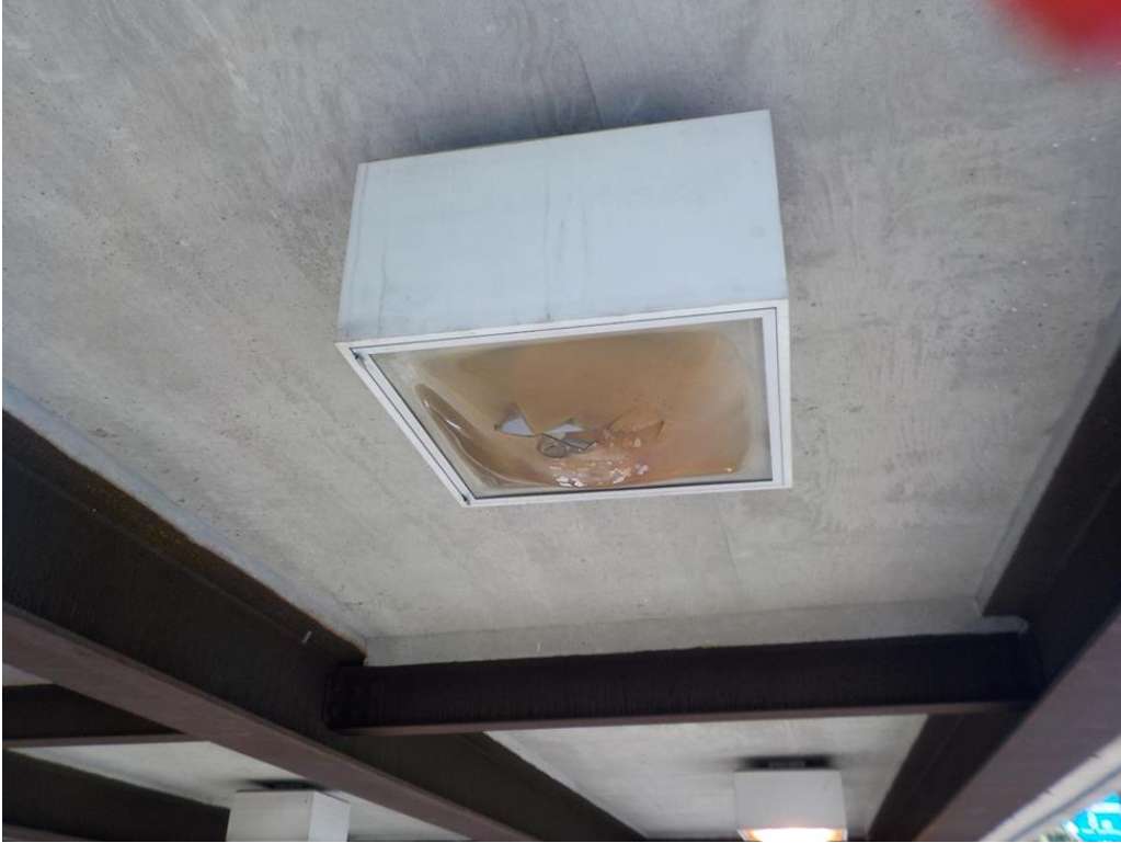
Photo 13: Cracked overhead light mounted to underside of slab.
