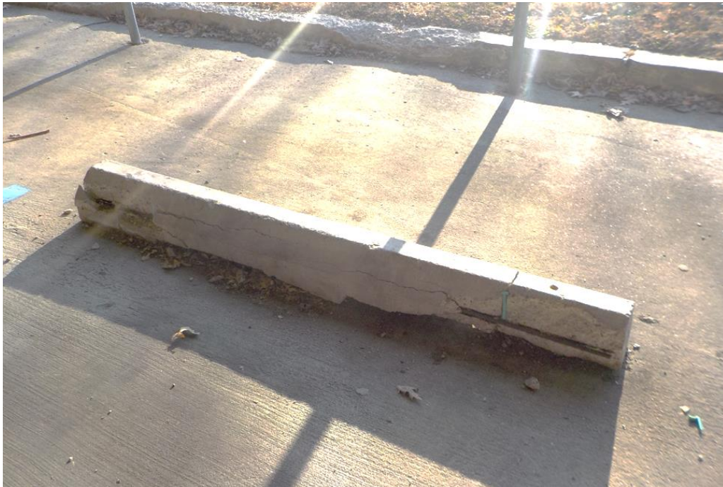
Photo 10: Spalled concrete wheel stop along south elevation.
