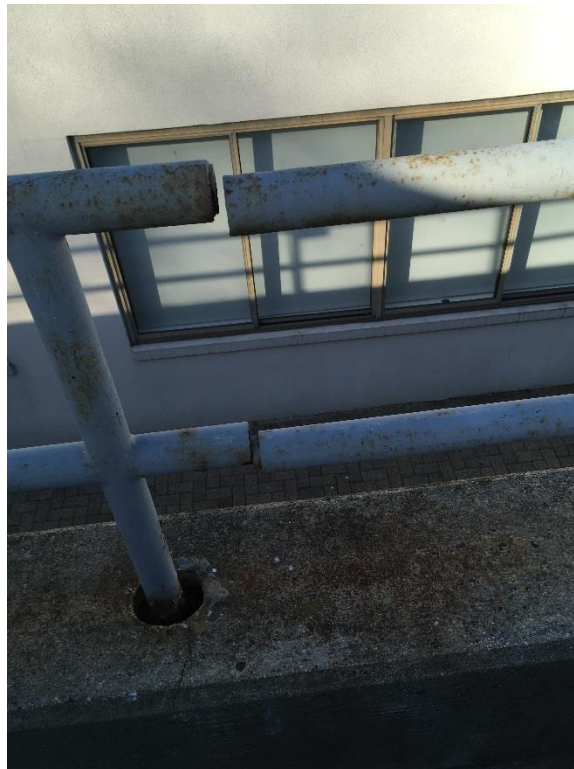
Photo 18: Deteriorated rail connection. Photo taken along north elevation.
