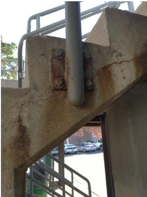
Photo 16: Corroded rail post connections anchored to distressed concrete. (L) south stair, (R) north stair.
