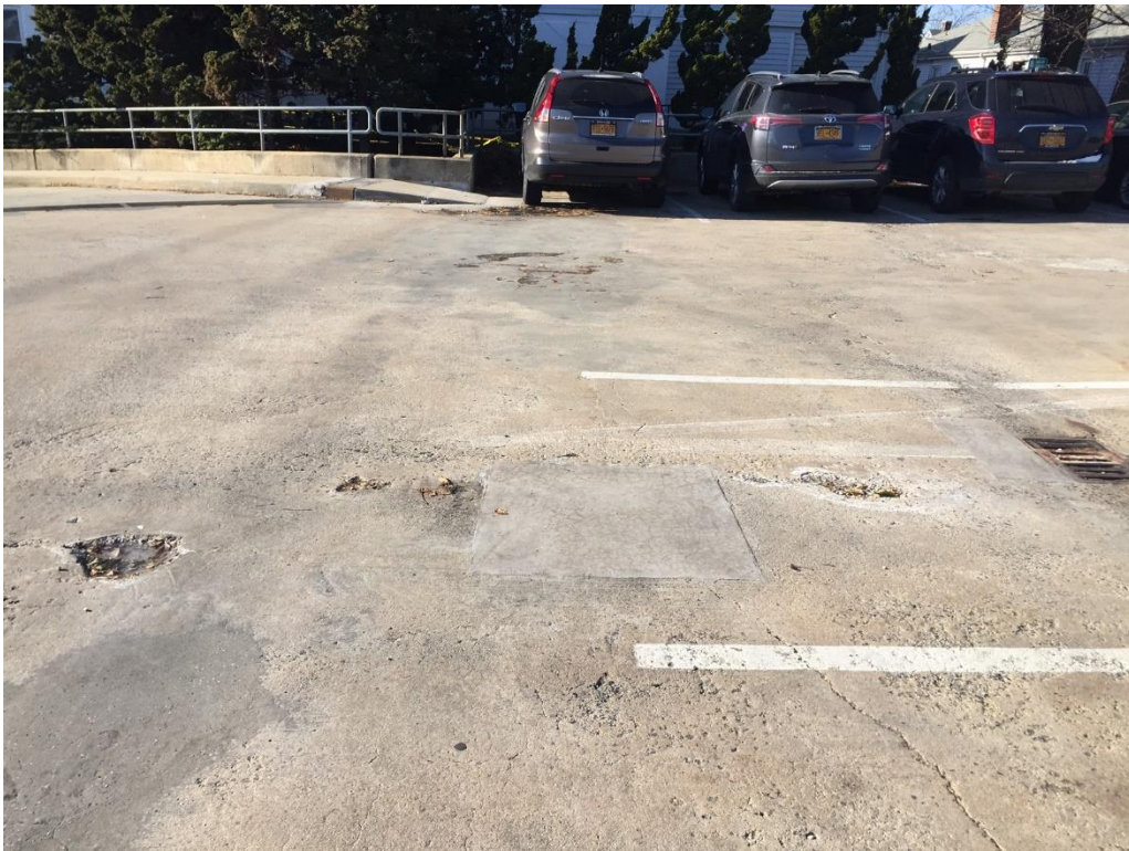
Photo 6: Spalls, concrete scaling, cracks, and ponded water at topside of slab. Photo taken south of the expansion joint.
