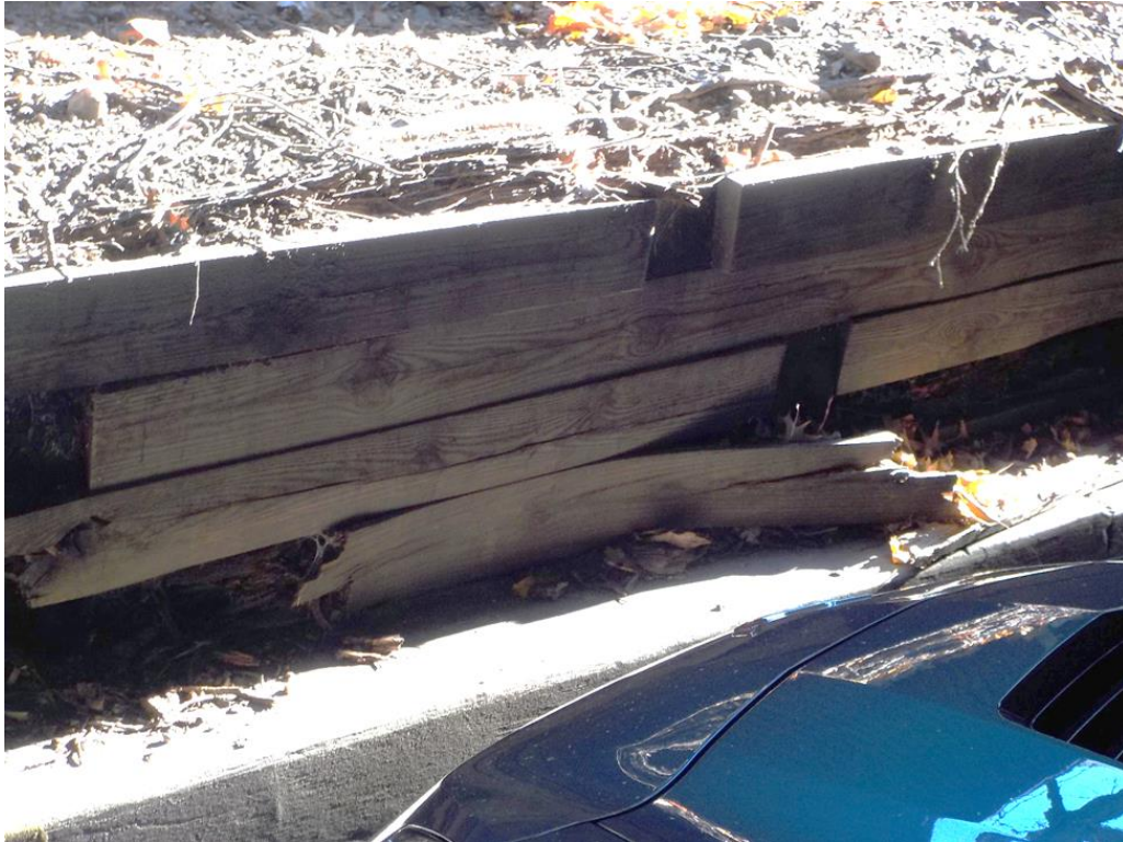
Photo 15: Deteriorated timber-tie wall along east elevation.
