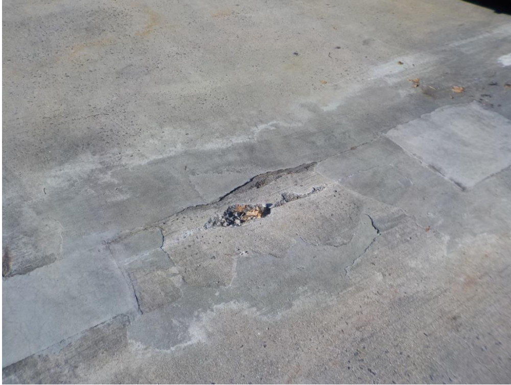
Photo 5: Spall at topside of slab. Photo taken south of the expansion joint.
