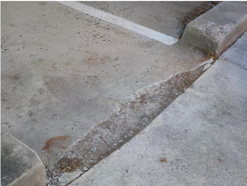
Photo 4: Spall in slab on grade. Photo taken at north elevation pedestrian entrance.
