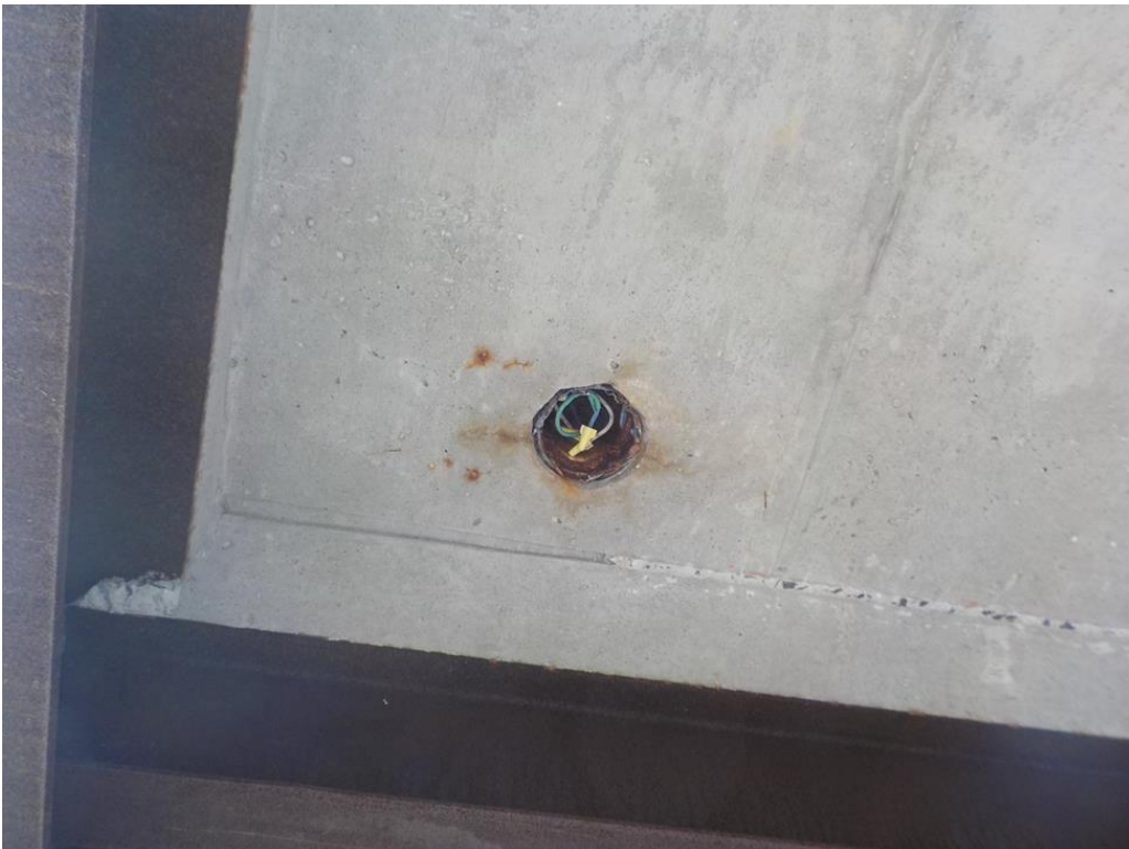
Photo 14: Exposed overhead electrical box.
