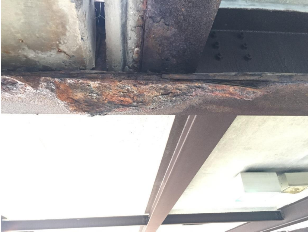
Photo 3: Loose rust at steel beam. Photo taken by south stair.
