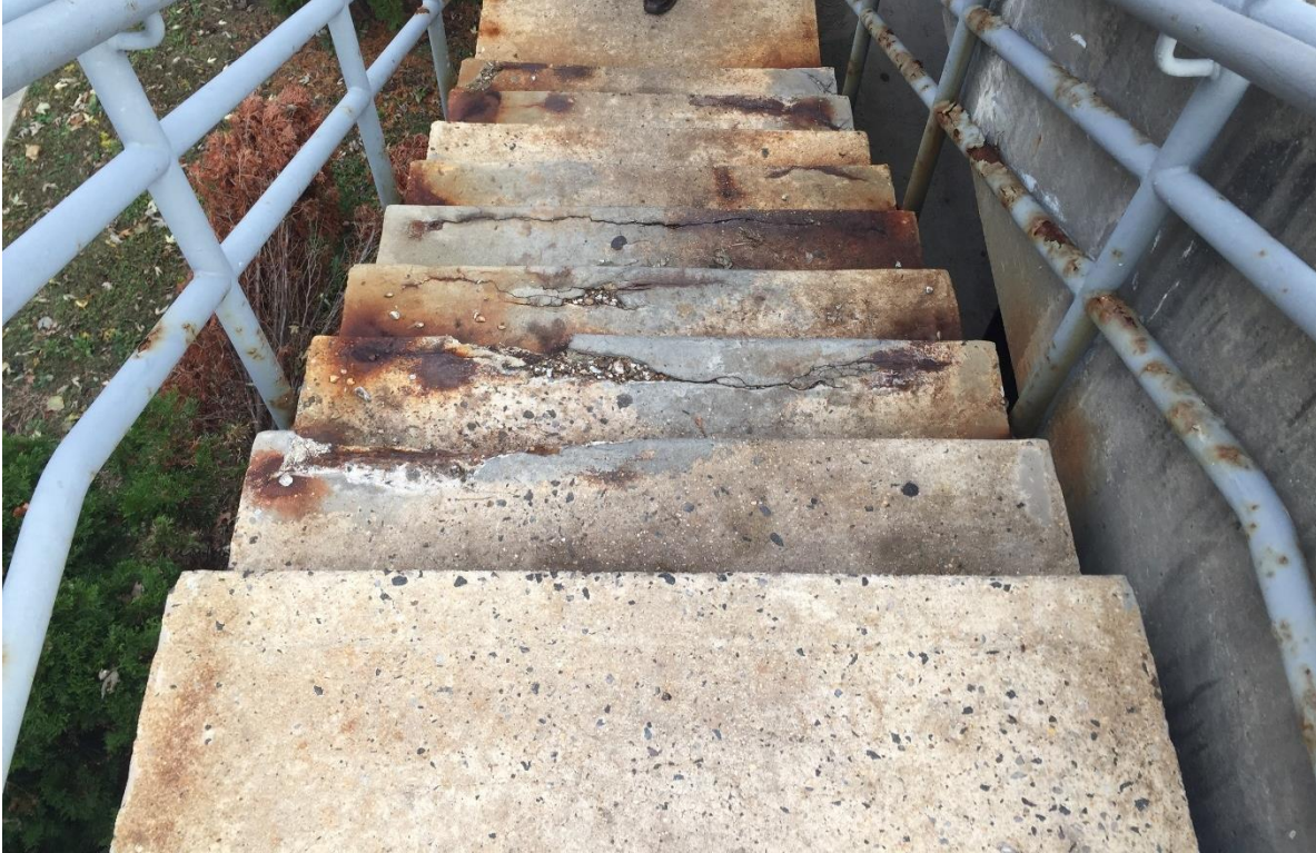
Photo 7: Spalls and cracks in stairs. Photo taken at north stair.
