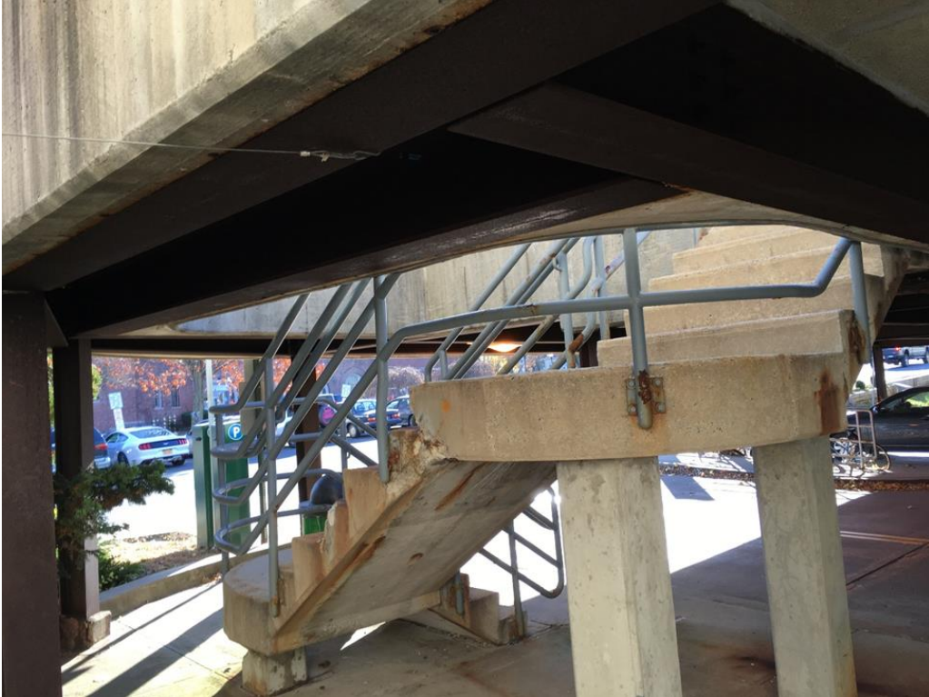
Photo 17: Gaps at stair railing greater than 4". Photo taken at south stair.
