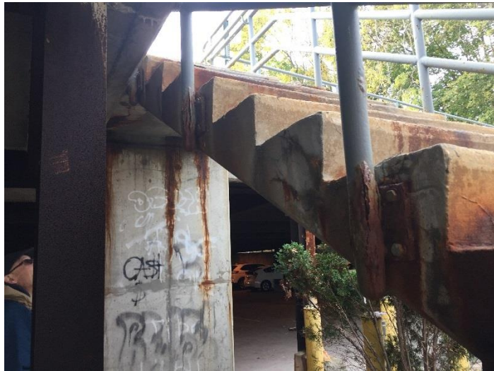
Photo 16: Corroded rail post connections anchored to distressed concrete. (L) south stair, (R) north stair.
