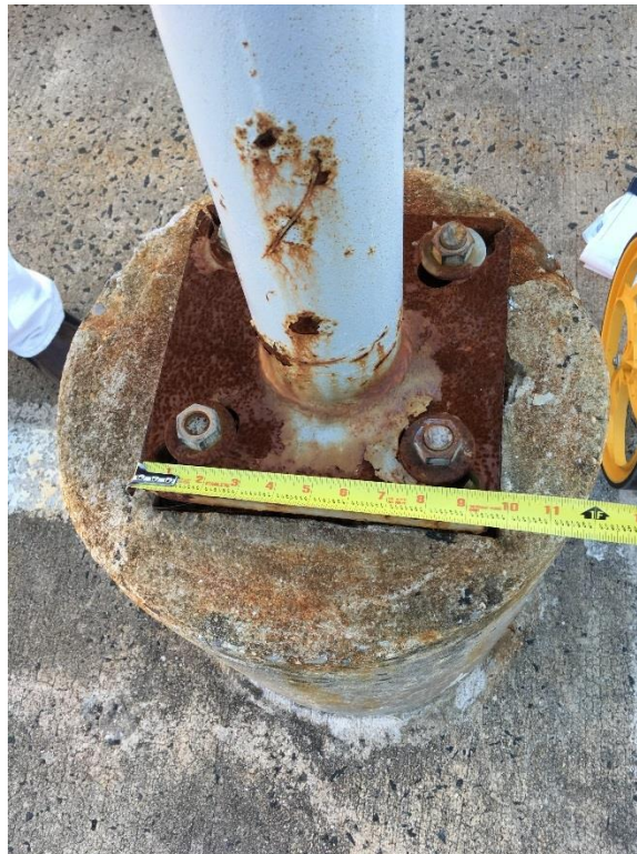
Photo 12: Corroded bolts. Photo taken at top parking deck light post.
