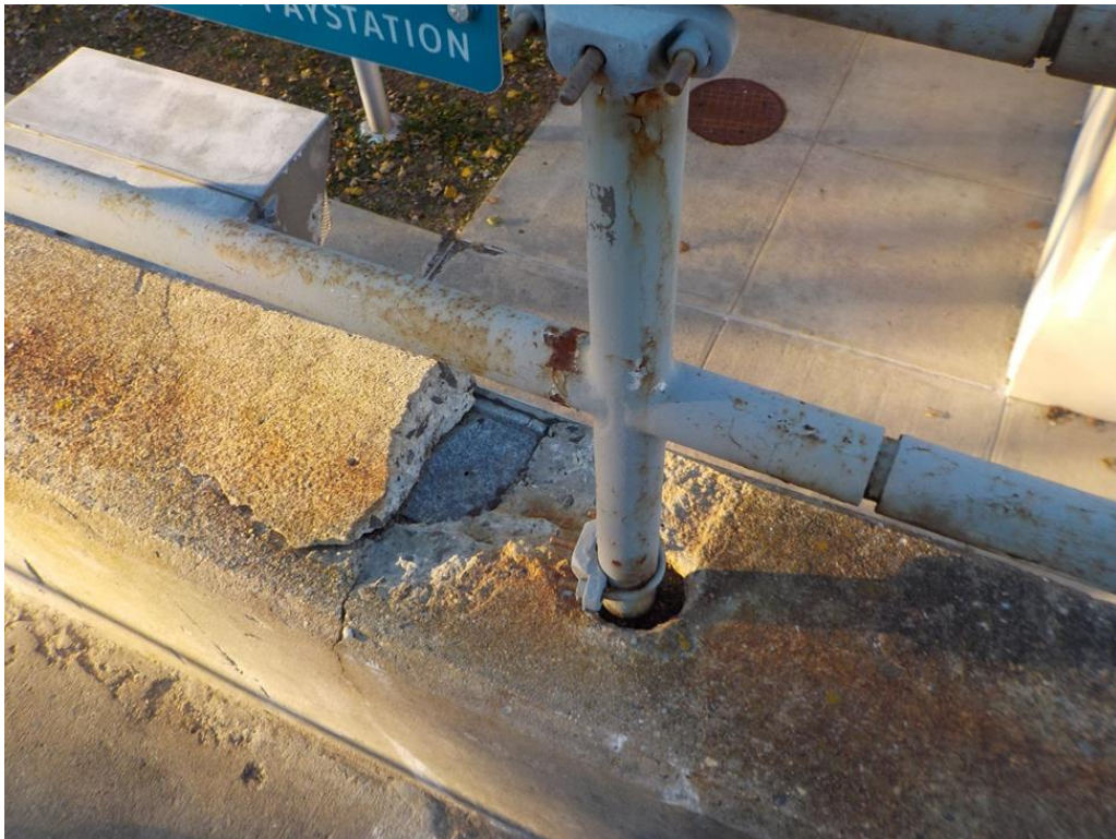
Photo 2: Loose concrete at parapet. Photo taken along north elevation.
