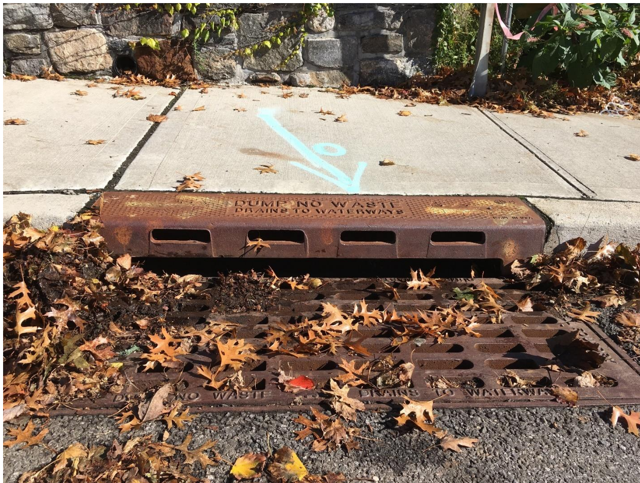
Figure 6 Example of a Type N catch basin designed to minimize storm sewer infiltration. Photo Credit: Matt da Silva
